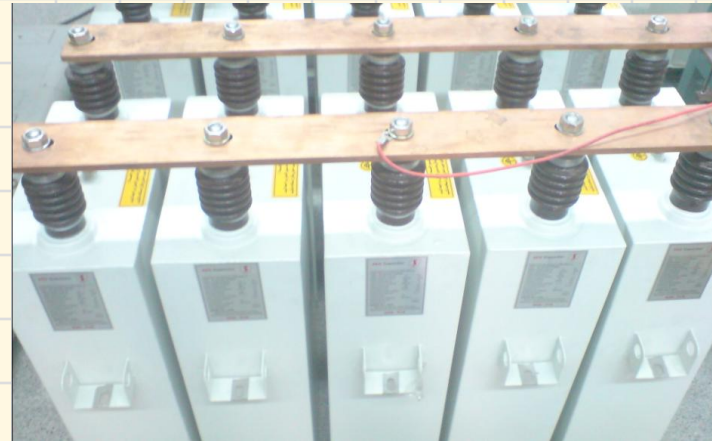
5 parallel 500 [uF] capacitor bank
